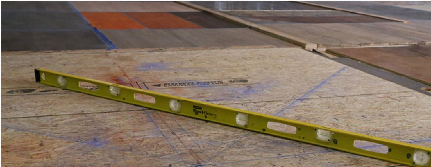
The subfloor is the foundation for the wood floor. Whatever happens below, will undoubtedly affect what's on top. In other words, an improperly prepared or inadequate subfloor will adversely affect how the wood floor performs. Subfloor flatness is one of the many considerations that should be addressed before installation of any wood floor.
